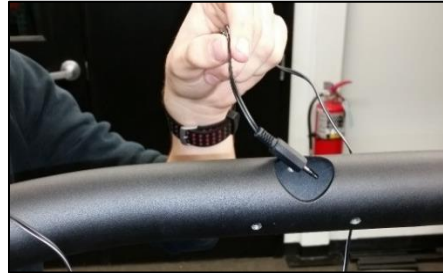
Fig. 9 Installation step, feed Data wire into horse-shoe
