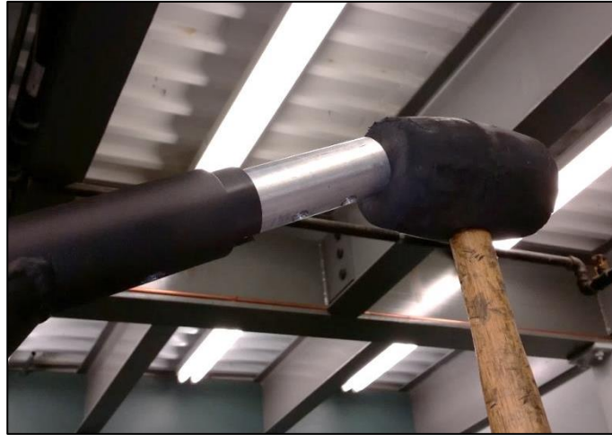
Fig. 15 Installing couplers (2)
